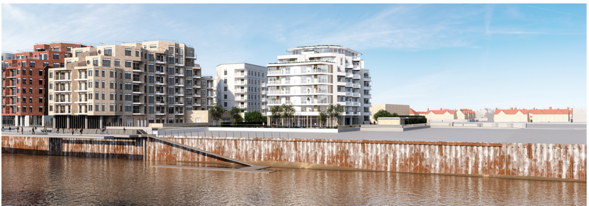
Figure 2 - Image of the development from riverside and Free Wharf to the west
